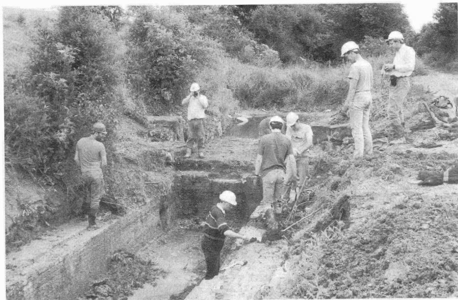
LWRG working on Moredon Bottom Lock, North Wilts Branch of the Wilts & Berks Canal PHOTO : Alison Smedley
